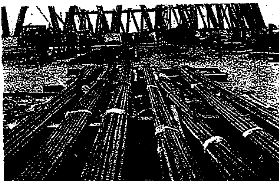
Coated Bars Stored At Job Site
