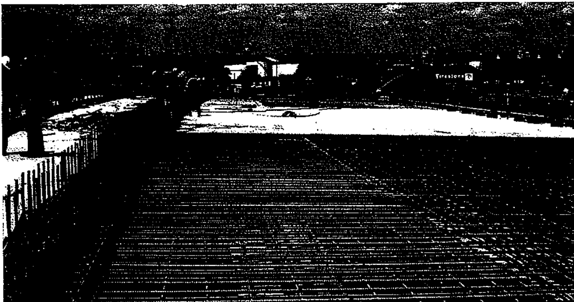
Coated Bars Placed In Bridge Deck Ready For Concrete Pour
