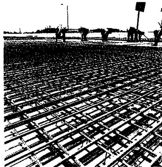
Iron Workers Completing Placement of Coated Bars In Large Bridge Deck
